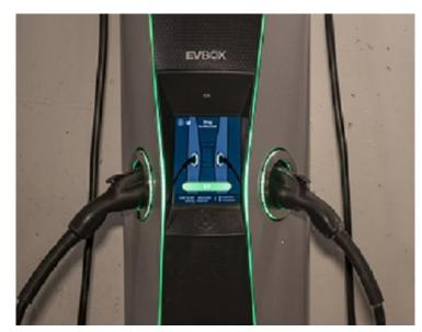
stations. Each of the 10 level 2 charging plugs in the underground garage can power a vehicle in about six hours.
